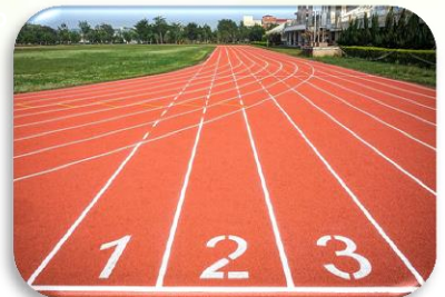
Base Layer for Running Track
